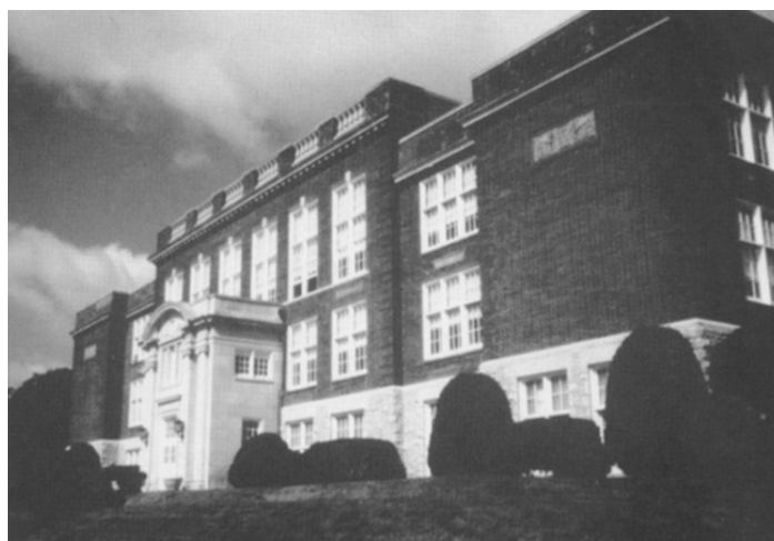
McClain High School, Greenfield, Ohio. (Photo by Virginia E. McCormick.)
