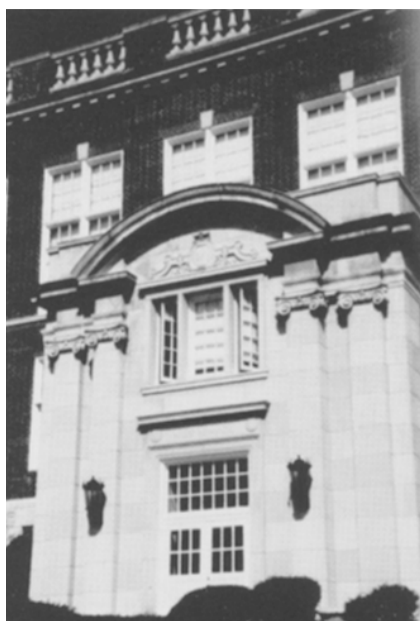
The entry is framed by pilasters and a semi-circular pediment displaying a cartouche. (Photo by Virginia E. McCormick.)
